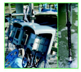
Conductivity is a well recognized, and sometimes indispensable, parameter of state-of-the-art water, wastewater and industrial process analysis. Continuous measuring systems are employed to monitor the salt load at the influent of wastewater treatment plants, to control quality of drinking water and ultra-pure water or to determine non-specific contaminants in industrial processes.
